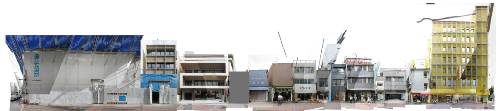
SS-16・19 SS-16・17 SN-15 SS-14 SS-13 SS-12 SS-11 SS-10 SS-9 SS-8 SS-7 SS-6
